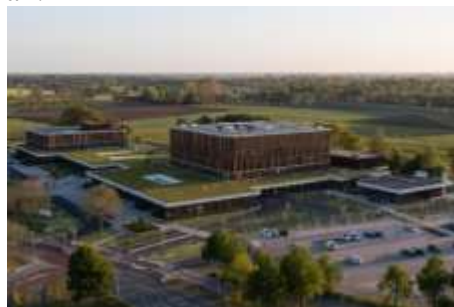
Gambar 1. Isala Meppel Hospital Sumber: Archdaily, 2022)
